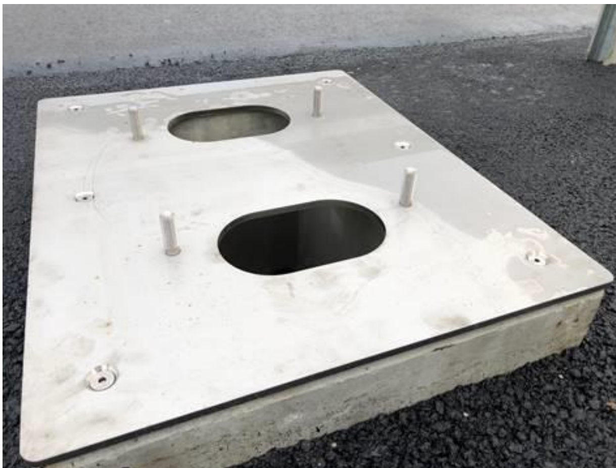
Top of a Unimi-1baseHPC foundation attached with an adaptor for a Tritium 150 kW rapid charger
